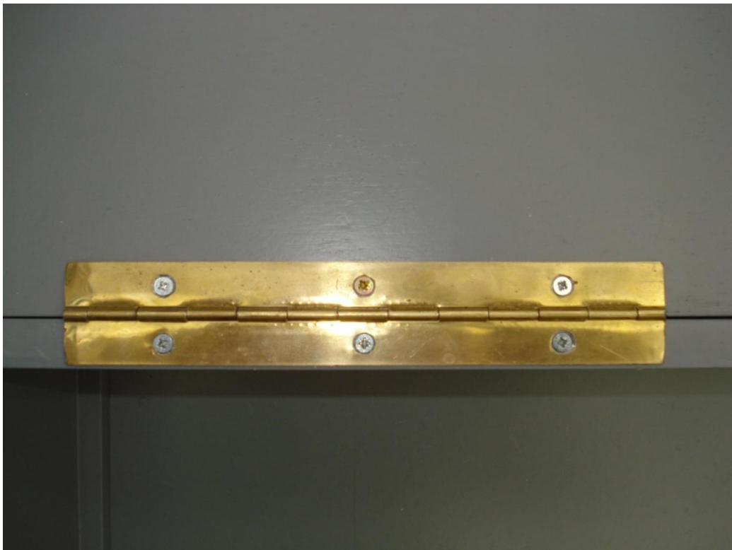
Figura 35 Bisagra de piano instalada
