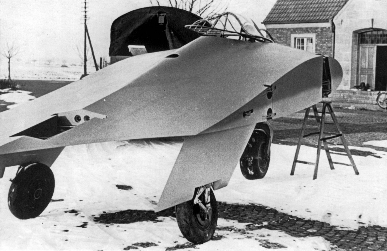
The center section of the H IX V1 at Göttingen before transport to the airfield. Visible in the photo above is the compartment for the aircraft's braking parachute.
